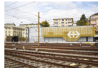
ENCLENCHEMENT CFF, LAUSANNE, 2017
