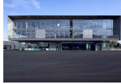
CENTRAL BUILDING, ORBE, 2006
