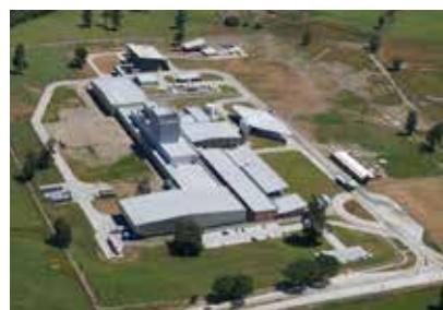
Nestlé Chile, Puelche (Chili) INDUSTRIAL BUILDINGS
