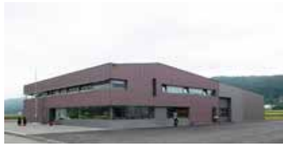
Despraz SA, Granges-Marnand (CH) INDUSTRIAL BUILDINGS
