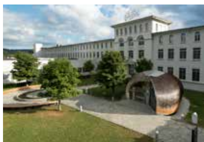
CCE Broc and Maison Cailler pavillion, Broc (CH) RESEARCH CENTRES
