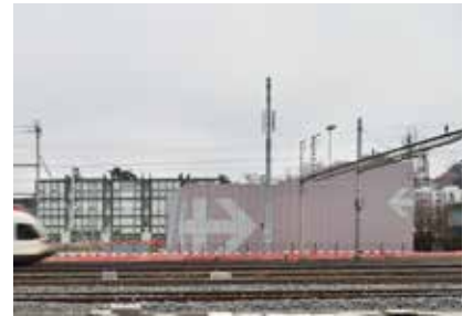
CFF service building, Renens (CH) INDUSTRIAL BUILDINGS
