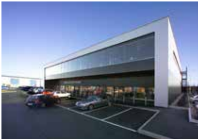
Commercial Center, Allaman (CH) COMMERCIAL BUILDINGS
