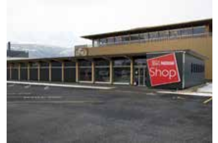
Nestlé Shop, Orbe (CH) COMMERCIAL BUILDINGS
